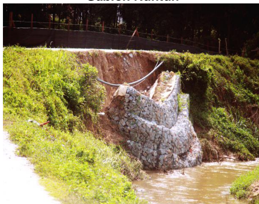
Gambar 1.8 Gabion Runtuh
